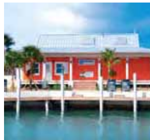
Phase I :: Scotts Landing Marine fuel Station features ValvTect Gasoline & Diesel
