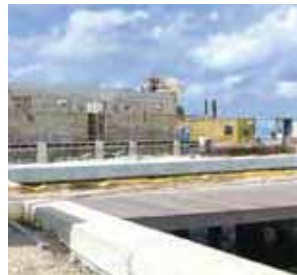
Phase I :: changing room with showers and lockers
